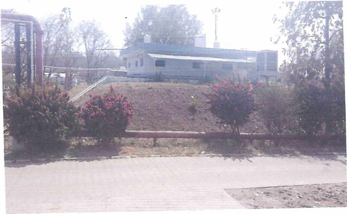
Photograph: South side process Building at the incident site
