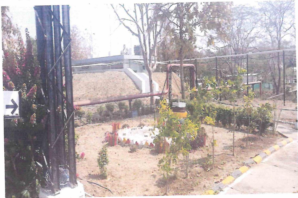
Photograph: South-West side process Building at the incident site
