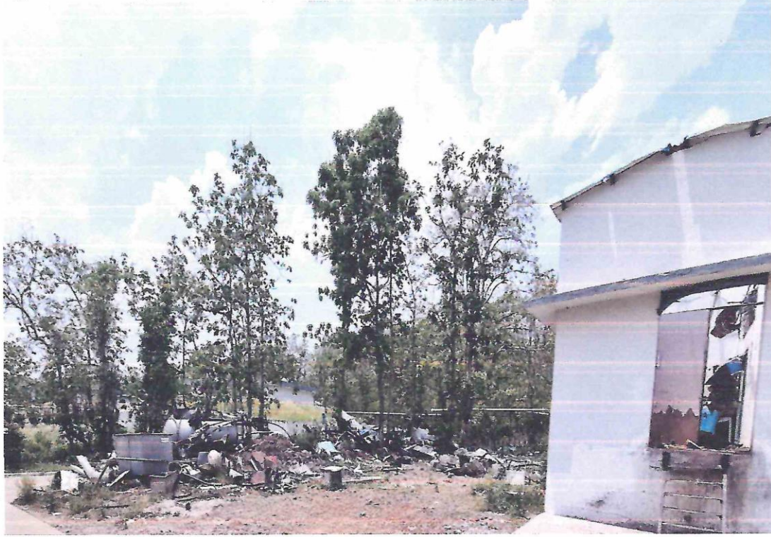
Fig: Photo of Utility shed attached to HR-CPCH-2 Building & Removed Damage Equipment
